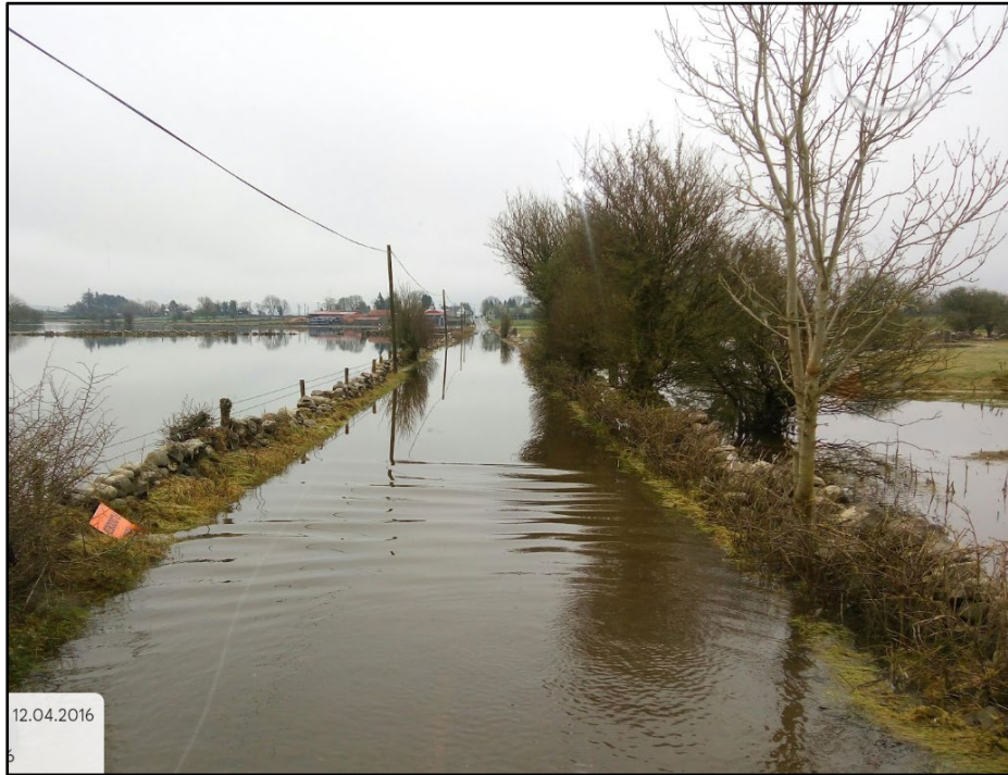
Photo 11: The R363 flooding looking south April 2016.
