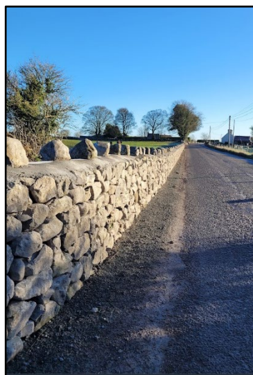
Photo 13: Finished retaining wall.
