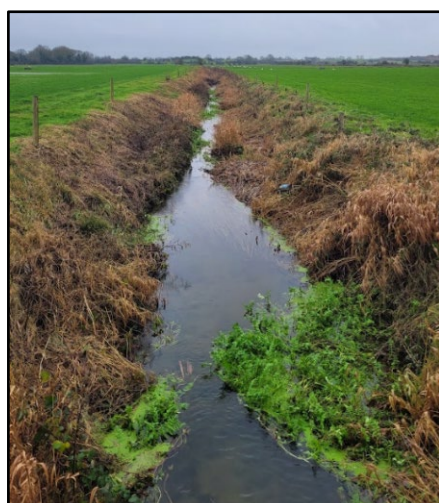
Photo 14: Culvert at L2023 Looking SE
