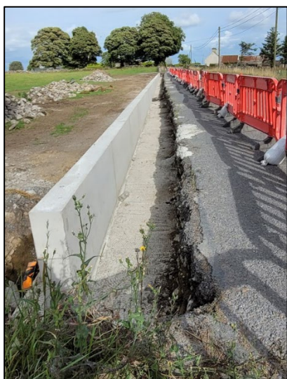
Photo 12: Retaining wall at the R363
