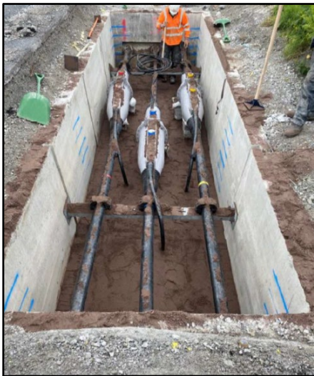
Figure 14a: Typical Joint Bay Backfilling Procedure
