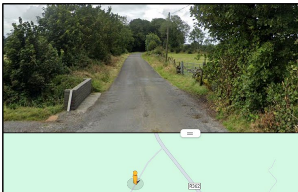
Photo No.5 drain culverted under L7720
