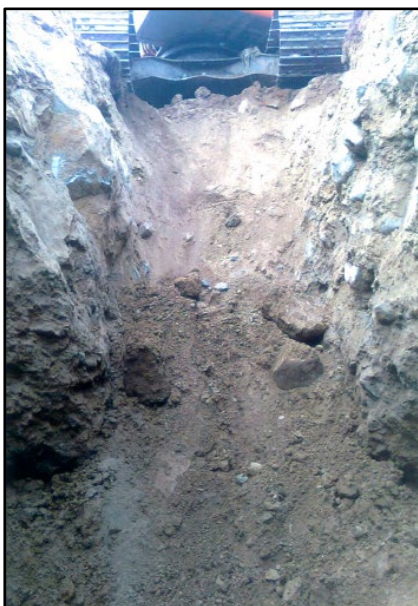
Photo 1: Collapsed subsoil
