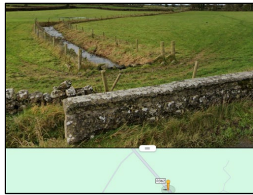
Photo No.6 drain culverted under the R362
