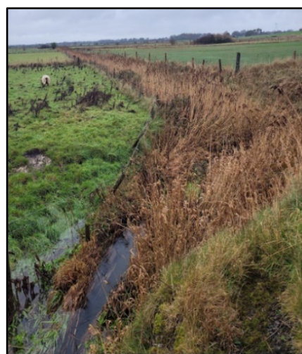
Photo 15: Culvert at L2023 Looking NW
